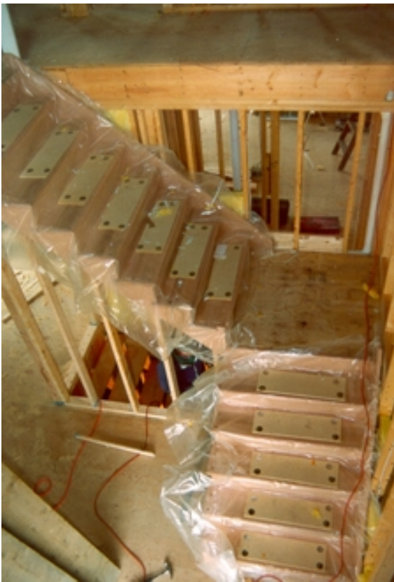
14 Riser “L” shaped stair set in rough, wrapped in plastic
